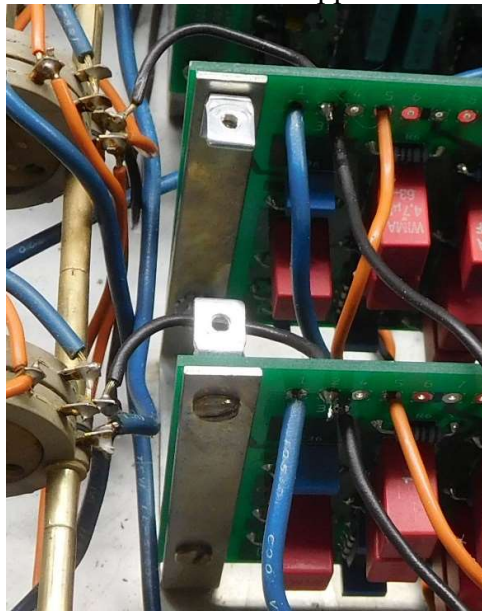
Figure 4-Replacing nuts with mounting brackets
